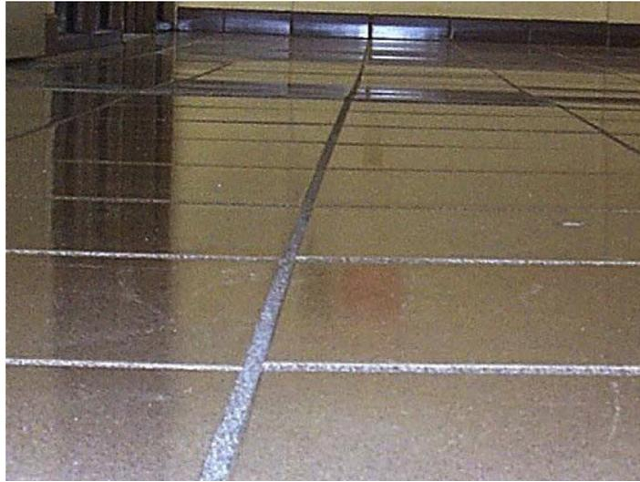
Picture 1-1 – Large format tile highlight imperfections in the substrate.
