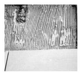
Picture 1.3 — Insufficient thin set adhesive coverage. Removal of a tile reveals many voids that are present in the hardened thin set adhesive Trowel ribbons are inconsistent which will also lead to poor coverage and adhesive transfer to the backs of the tiles.
