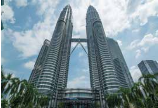
1999 – PETRONAS TWIN TOWERS, KUALA LUMPUR, MALÁSIA
