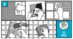
Apply mortar to the substrate with the flat side of the trowel, pressing firmly to work into surface. Comb on additional mortar with the notched side.
