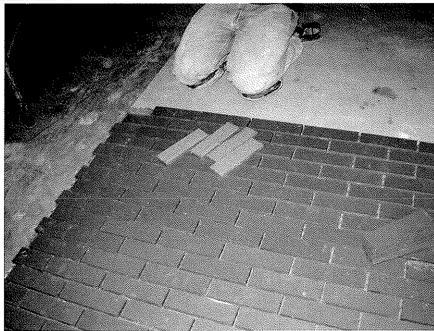
Masonry application on to test frame
