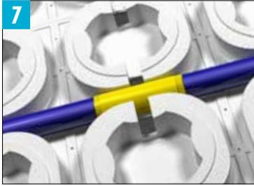
STRATA\_HEAT Wire is manufactured so that there is a spliceless connection where the heating cable meets the coldtail. **This connection is marked with tape and MUST be installed within the STRATA\_HEAT Mat and covered with adhesive and not exposed.** Ensure this connection is installed straight in the STRATA\_HEAT Mat and not bent around a peg.
