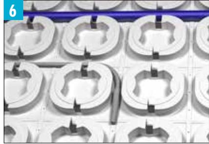
Install the floor sensor at least 6" (15 cm) into the heated area it will be controlling. It should be located centrally between parallel runs of heating cable and not in an area influenced by other heat sources.
