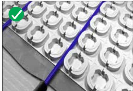
STRATA\_HEAT Wire cannot be installed across expansion joints within the floor. Where a heated floor is divided by expansion joints, individual wires should be used to heat each area. The cold tail may cross the expansion joint within a 12" (30 cm) long UL/cUL certified conduit if necessary.
