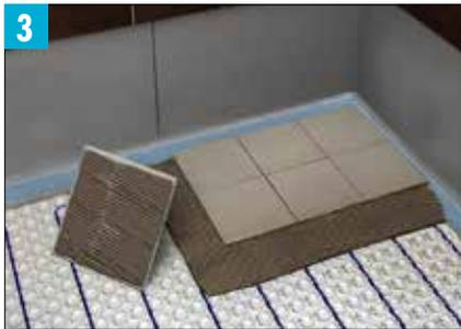
After laying the first tile remove and ensure the tile is getting a full coverage of adhesive from your application.
