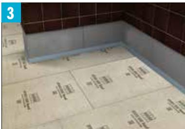
(Optional) Install expansion strips along any perimeter or sectional expansion joints within the subfloor to preserve their function.
