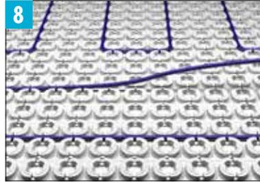
Install the STRATA\_HEAT™ Wire at the chosen spacing. Maintain a minimum 3 peg (2 3/8" / 60 mm) spacing for UL Compliance. Install the floor sensor centrally between two runs of the heater wires. For the termination joint, channel a groove in the STRATA\_HEAT Mat, enabling the joint to fit flush with the top of the mat. DO NOT tape over the termination joint.
