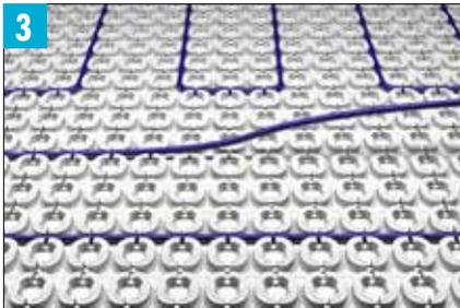
Begin laying the STRATA\_HEAT Wire, pressing it between the pegs. Maintain proper spacing and make sure the heating wire doesn't cross itself.
