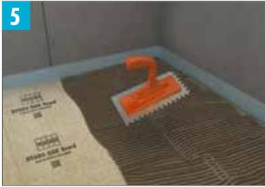
Apply a thin-set layer to the substrate using a ¼" x ¼" (6 mm x 6 mm) square notch trowel.
