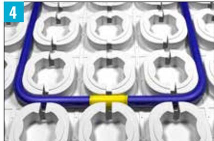
The STRATA\_HEAT™ Wire has a marker at its midpoint. When you reach it, review your progress up to that point and check that you are correctly spacing the wire, ensuring that you will have covered the whole of the heated area when you reach the end of the wire.
