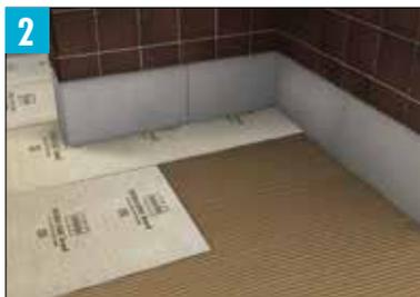
Recommended Step - Install HYDRO BAN® Boards for insulation over the subfloor referring to DS-040.0 installation instructions.
