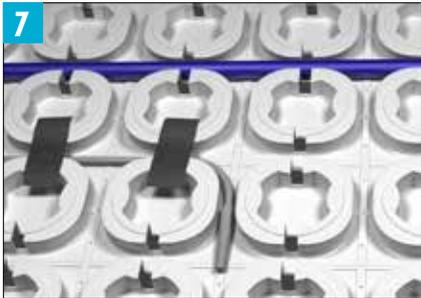
Measure the resistance of the floor sensor and record it on the control card on Page 32. If its resistance is outside the prescribed range contact our technical helpline.
