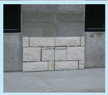
Adhered veneer installation with MVIS™
