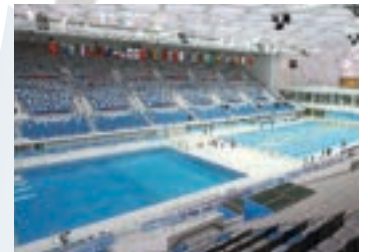
Beijing National Aquatics Centre | Beijing, China
