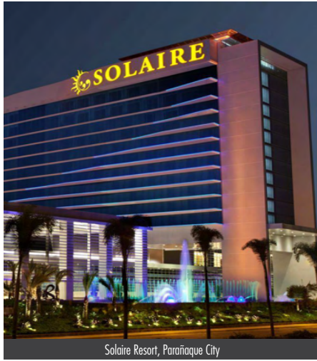
Solaire Resort, Parañaque City
