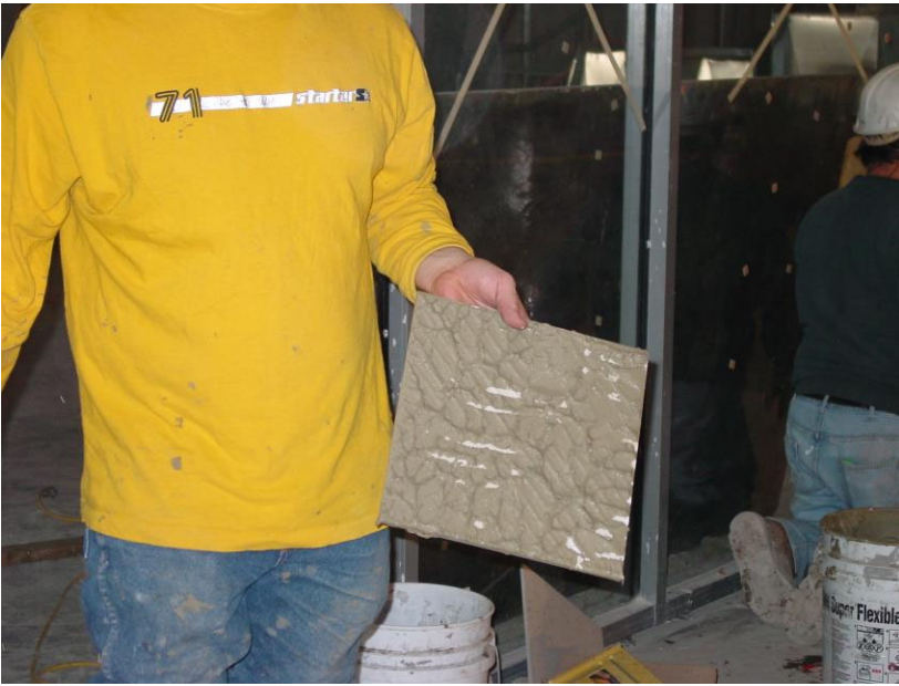
Picture 1.4 – Ceramic tile removed during the installation to verify proper coverage is being attained. Notice the lower right hand corner of the tile is lacking coverage. This will undoubtedly lead to a cracked tile.
