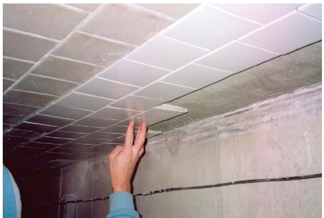
Figure 8.1 — Installation of Exterior Rated Ceramic Wall Tiles on the Ceiling of the Route 9A, New York, NY Roadway Tunnel Utilizing the Epoxy Spot Method — LATAPOXY® 310 Stone Adhesive
