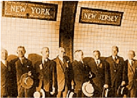
Figure 5.5 – Holland Tunnel Dedication, November 12, 1927. Notice the ceramic tile clad walls and the ceramic mosaic tiles state murals. Photo courtesy of the Port Authority of New York and New Jersey.
