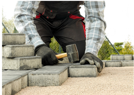
Figure 4.2 – Sand Set Pavers
