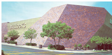
Figure 7.1 — High adhesive shear and tensile strength to resist seismic movement. Before photograph of the Bullock's building prior to the Northridge, CA earthquake in 1994. Tiles were installed on the exterior façade with 4237 Latex Additive mixed with 211 Powder over 9235 Waterproofing Membrane.
