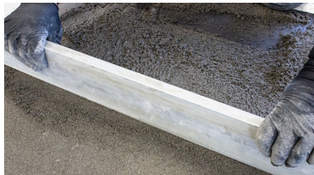
Figure 2.9 — Installation of an unbonded wire reinforced mortar bed.
