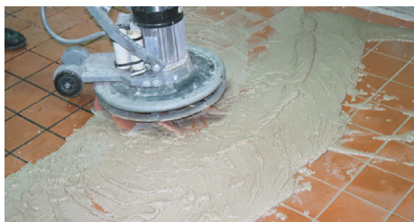
Figure 8.24 – Grout Spreading Process.
