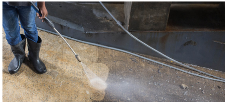
Figure 3.2 – High-pressure water washing.
