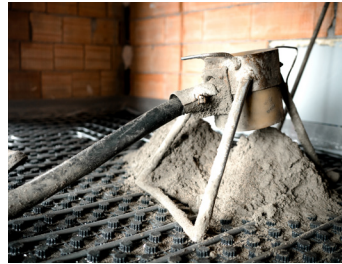
Fig. 8.22 – Mortar Mixer and Pump.
