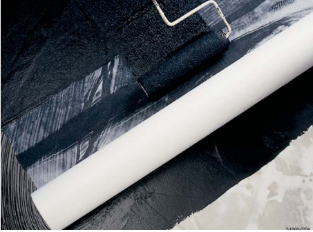
Figure 6.2 – Liquid applied membrane applied to concrete substrate.
