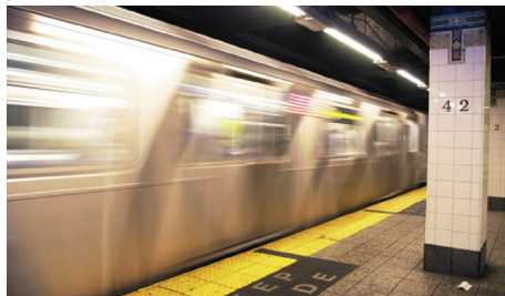
Figure 8.25 – Restoration of the 42 nd Street Subway Station, New York, NY. Granite pavers installed with LATICRETE® 211 Powder mixed with LATICRETE 4237 Latex Additive over a mortar bed consisting of LATICRETE 226 Thick Bed Mortar mixed with LATICRETE 3701 Mortar Admix. Installation by Navillus Contracting Inc., Long Island City, NY.
