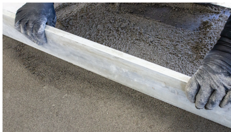
Figure 7.13 – Tile mechanic screeding a mortar bed.
