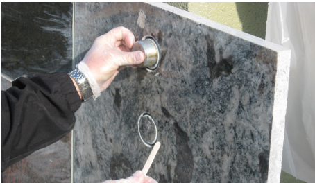
Figure 9.6 – Metal disc is held or mounted in place until epoxy resin is cured.
