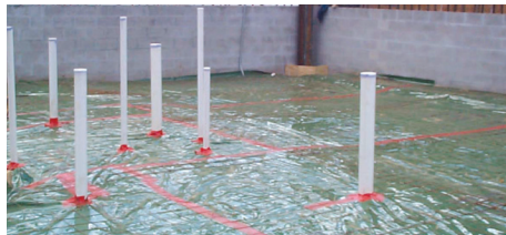
Figure 2.13 –Proper vapor retarder placement.
