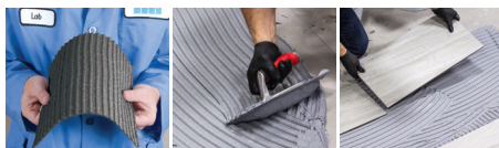
Figure 6.1 — Trowel applied sound and crack adhesive mortar applied to concrete substrate.
