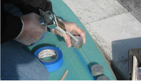
Figure 9.5 – 2" (50 mm) diameter metal disc to be adhered to the stone surface with a two component epoxy resin adhesive.
