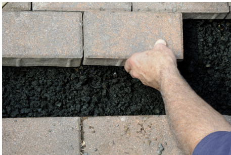
Figure 4.3 – Bituminous Set Pavers
