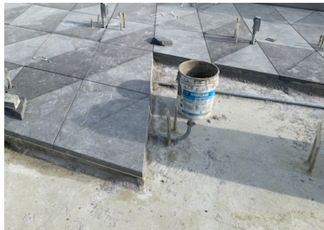
Figure 4.4 – Mortar Set Pavers
