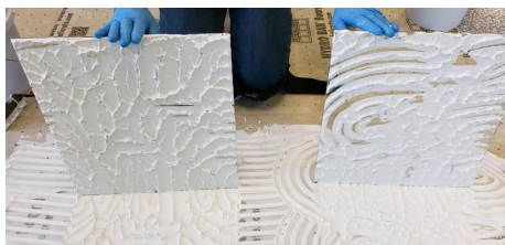
Figure 8.15 — Examples of incomplete bedding due to lack of sufficient mortar and/or incorrect trowel size selection and beat-in.
