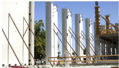
Figure 3.1 — Tilt Up Concrete Panels erected into place. Photo courtesy of www.constructionphotographs.com .
