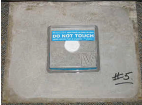
Figure 2.18 – Calcium chloride test in place (Photo Courtesy of Vaprecision).
