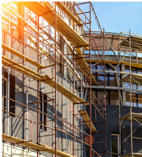
Figure 8.3— Example of tubular scaffolding.
