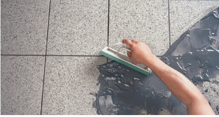
Figure 7.23 – Spreading of Epoxy Grout.
