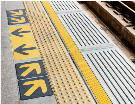
Figure 5.6 – Tile Installation with Warning Tile at a train platform.
