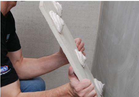
Figure 7.18 – Stones are then placed, leveled and plumbed to the required finish.
