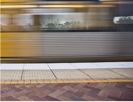
Figure 5.7 – Klinker tile at a train platform.
