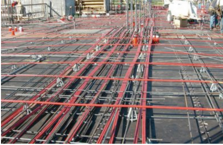
Fig. 2.22 – Post tensioned concrete slab. Notice the orange tensioning cables that will run throughout the concrete slab. Photo Courtesy of SunCoast Post Tensioning Company.
