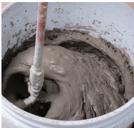
Figure 7.3 — Mixing of liquid latex fortified portland cement medium bed mortar.
