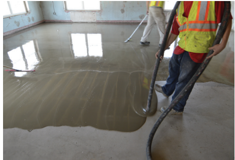
Figure 7.19 – Application of self leveling underlayment over a primed concrete substrate.
