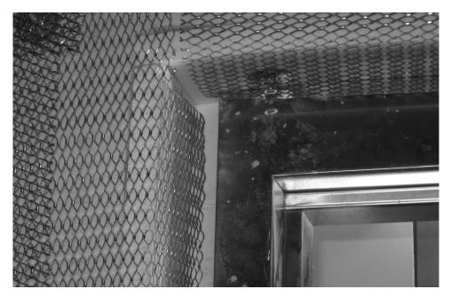
Installation of 3.2# expandable diamond metal lath to stainless steel door frame and flashing.
