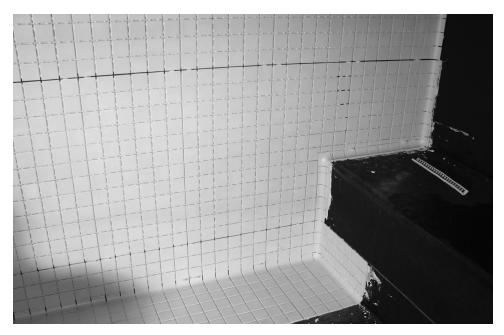
Installation of tile onto 9235 Waterproofing Membrane using 254 Platinum.
