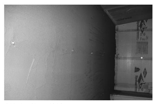
A finished scratch coat wall that is now ready for the float coat.
