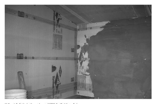
Wall partially finished with scratch coat of 3701 Fortified Mortar Bed.
