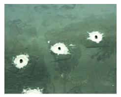
Figure 6.3.5 — Epoxy waterproofing membrane is applied at the pipe penetrations over the cured liquid applied waterproofing membrane to ensure a complete seal at the penetrations.
