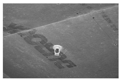
Ceiling (with fire sprinkler head) showing Tile Council of North America (TCNA) recommended pitch of 2" per foot (50mm per 300mm).
