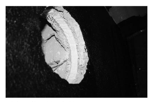
Scratching the 3701 Fortified Mortar Bed with a piece of metal lath.
