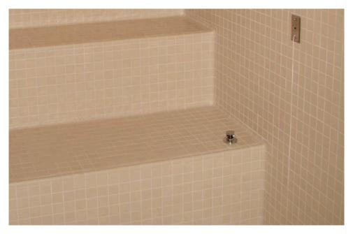
Same view of finished installation after grouting with SPECTRALOCK® PRO Premium Grout and LATASIL $^{\mathbb{M}}$ .
