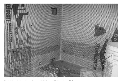
Bench/wall transition and proper placement of 3.2# expandable diamond metal lath.
