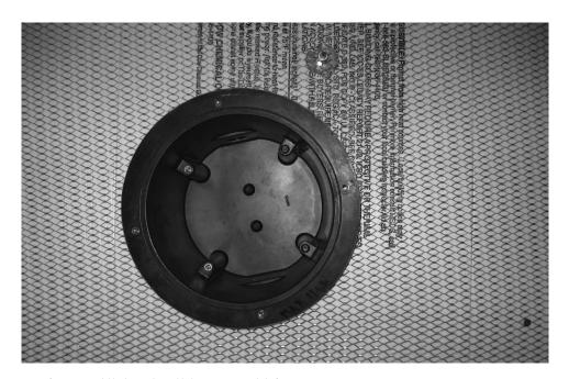
Tie-in of 3.2# expandable diamond metal lath to steam room light fixture.
