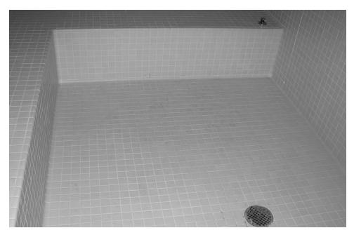
Finished floor installation of tile. Floor and seats are sloped  $\frac{1}{4}$ " per foot (6mm per 300mm) to the drain.
