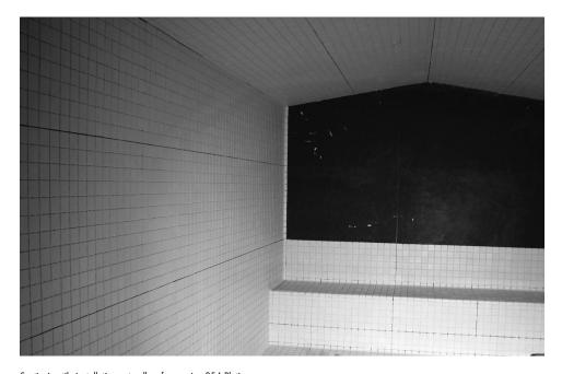
Continuing tile installation onto all surfaces using 254 Platinum.
