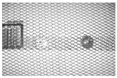
3.2# expandable diamond metal lath fastened through the rigid foam insulation board that has been installed over a vapor diffusion retarder (vapor barrier).
