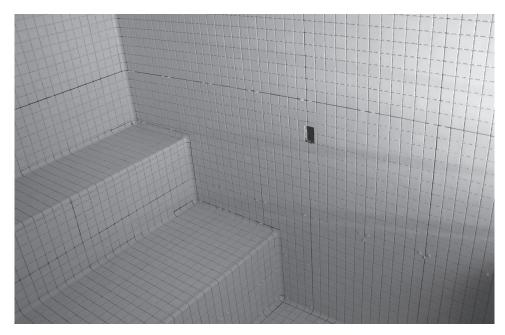
Finished installation of 2" x 2" (50mm x 50mm) vitreous tile using 254 Platinum. Notice the cut-out in the wall for the emergency call switch.
