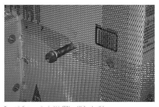
Pipe penetration for steam generation unit and tie-in of 3.2# expandable diamond metal lath.
