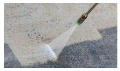
Figure 6.7 — High pressure water wash (water-blasting) may remove the required amount of contaminated concrete.
