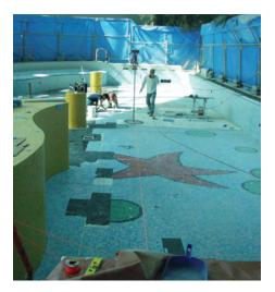
**Case Study 12** — The installation of the tile in the horizontal areas is now complete. Once the tiles are installed and grouted; the installation must cure for a full 14 days after the final grouting period at 70°F (21°C) if a latex fortified portland cement based grout (e.g. PERMACOLOR<sup>™</sup> Select Grout) is used or 10 days if an epoxy based grout (e.g. SPECTRALOCK<sup>®</sup> PRO Premium Grout\*) is used.
