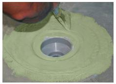
Figure 12.4 — The liquid applied waterproofing membrane must be flashed into a two part clamping style drain to create a watertight seal.
