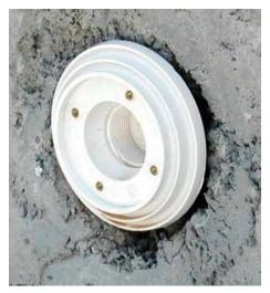
Figure 4.7 - Return port in a concrete shell pool8.
