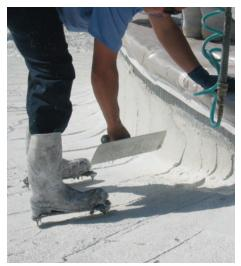
Figure 5.10 - Typical Marcite plaster installation (notice the spiked shoes).
