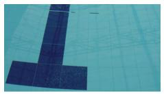
Figure 12.12 – Sealant in the movement joint is missing. In order for the sealant to maintain its functional ability, the joint must be correctly designed. Namely:
