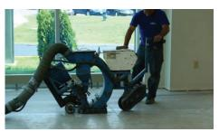
Figure 6.6 – Shot-blasting is ideal for areas outside of pool tanks and water features and for areas where access by the equipment is not an issue.
