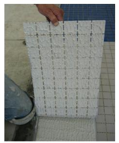
Figure 12.9 — It is good practice to periodically lift / remove freshly installed tiles or stones to verify that a minimum 95% continuous adhesive mortar is achieved. If the desired coverage is not achieved, use a larger trawel to dispense adequate adhesive mortar and beat-in the tiles correctly to achieve the desired results.
