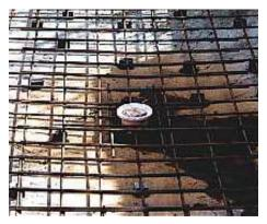
Figure 4.5 — Typical drain position and steel reinforcement prior to gunite application of concrete.
