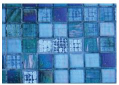
Figure 12.10 — The effects of a mesh mounted glass tile utilizing an adhesive and mesh that are not suitable for continuous submersion. The adhesive has expanded and last bond to the back of the tiles.
