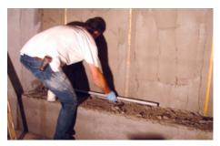
Figure 7.2 — Latex fortified render is being applied to wall surface. Notice the lath strips that are set into the mortar. The lath strips are leveled and plumbed to establish the correct wall render depth. Once the render achieves a sufficient cure, the lath strips are carefully removed and the cavities are filled with mortar.
