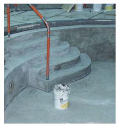
**Case Study 3** – The use of a LATICRETE<sup>®</sup> liquid latex fortified portland cement based leveling mortar is used to correct any irregularities in the concrete shell. Proper surface preparation will result in an aesthetically pleasing tile or stone finish.
