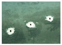
**Case Study 9** — The penetrations are sealed with a suitable flexible sealant. Generally, 100% silicone sealant (e.g. Latasil<sup>™</sup> with 9118 Primer) or urethane sealant with non-solvent based primers can be used. All precautions to create a complete watertight tank must be taken to ensure a successful flood test.
