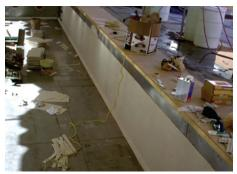
Figure 12.5 — Steel pool tank. Porcelain mosaic tiles are installed with a 100% solids epoxy thin set mortar adhesive (e.g. LATAPOXY® 300 Epoxy Adhesive) to achieve a suitable bond to the steel tank assembly.
