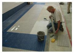
Figure 12.8 – Only enough latex fortified portland cement thin set mortar is spread to allow the installation of the porcelain mosaics within the mortar's typical open time – generally 15 minutes at 70°F (21°C).
