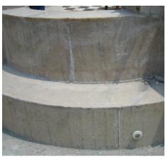
Figure 3.4 - A fiberglass pool shell waiting installation of tile.
