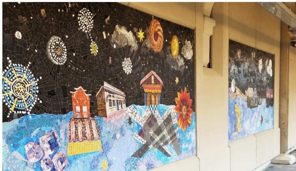
“Given the architectural requirements of these stations, we pre-mounted and grouted the designs on aluminum panels using products from LATICRETE, a prestigious brand leader in installation systems that we knew were tested and guaranteed for high-performance and ideal for exterior applications.”
